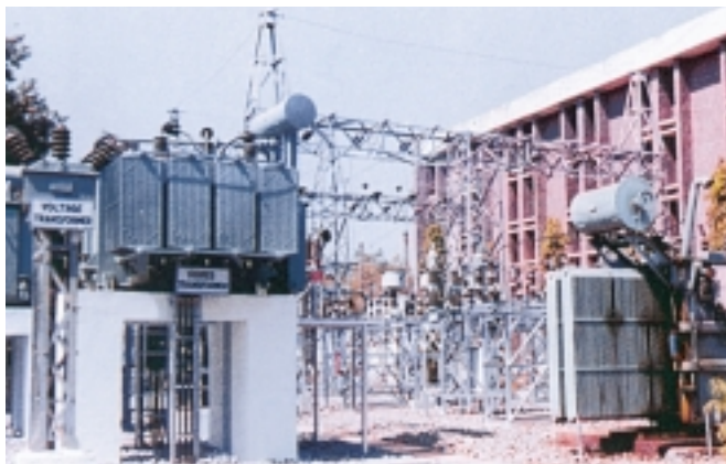
2 MVA Phase Shifting Transformer to enhance power transfer capability and improve system stability between two parallel 33 kv transmission lines - an innovation in the field of Flexible AC Transmission (FACTS)
