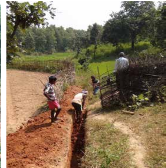
Excavation of trench for laying pipeline
