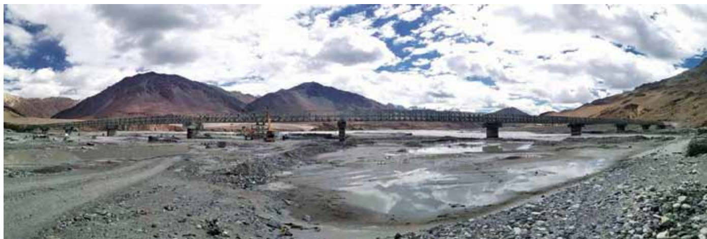
Manufacture, supply, erection and commissioning of 1400ft. (10x140') long Bailey Bridge of carriage way of 4.25m on Darbuk Shyok-Daulat Begh Oldie Road in Leh, for the Border Road Organisation
