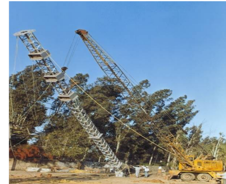
Emergency Restoration System (ERS)
