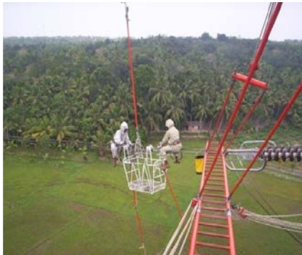
Hot Line Maintenance
