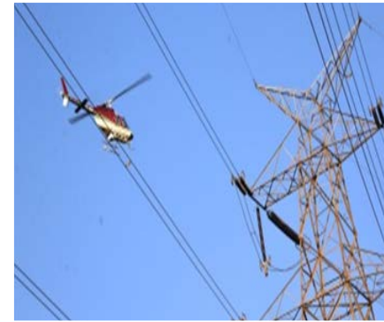
Aerial Patrolling using Helicopters
